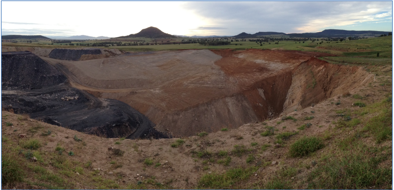
Plate 1 - Completed spontaneous combustion capping
